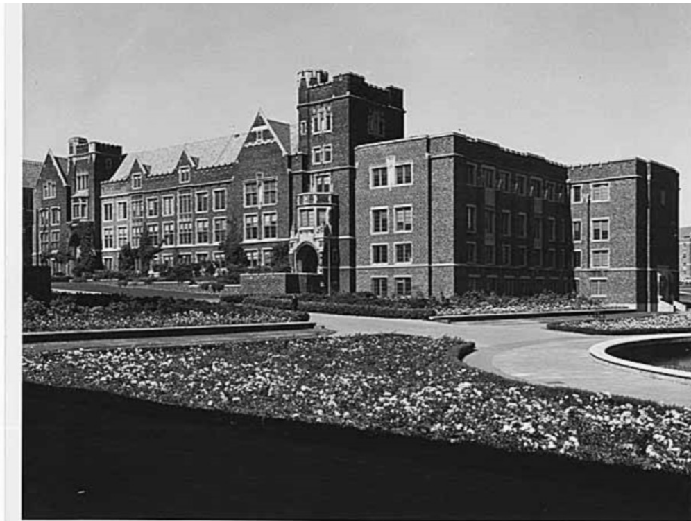
Figure 83. 1958 view of Physics Hall following the Carlson, Eley & Grevstad addition. University of Washington Libraries, Special Collections, Negative Number NIS(I)5074B.
