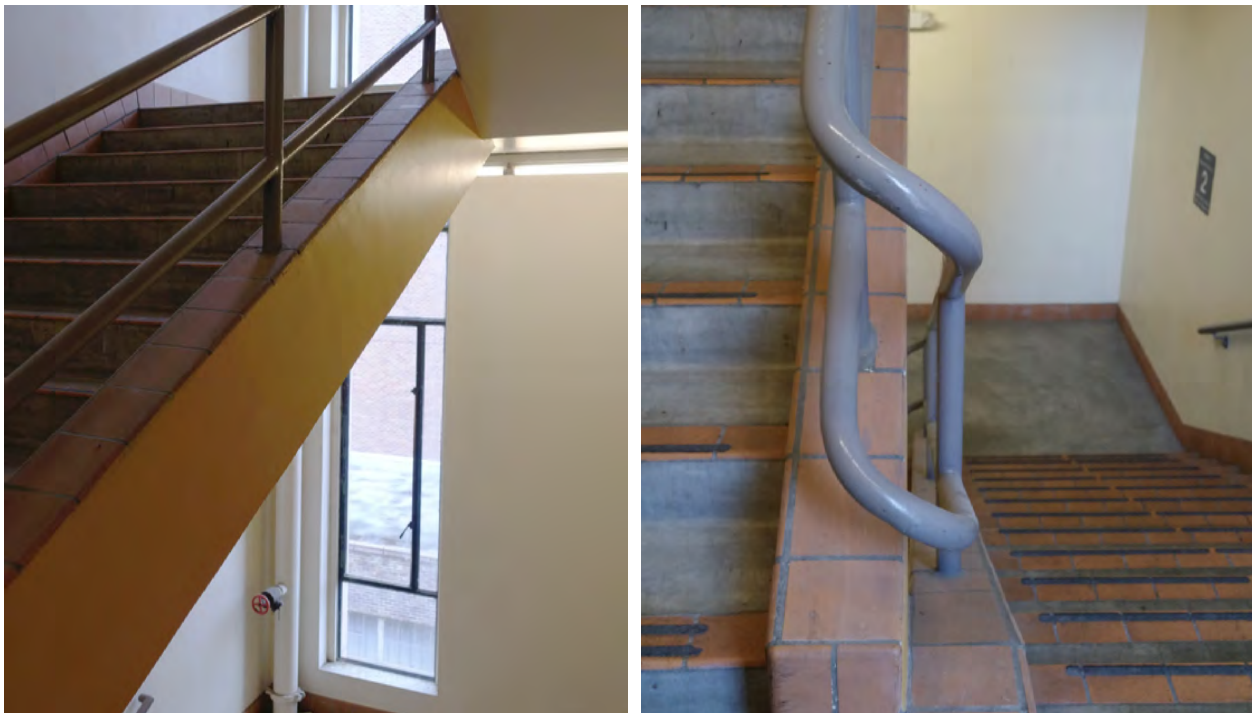
Figure 41. East stairwell, at the first story (above left), and stairwell detail (above right).
