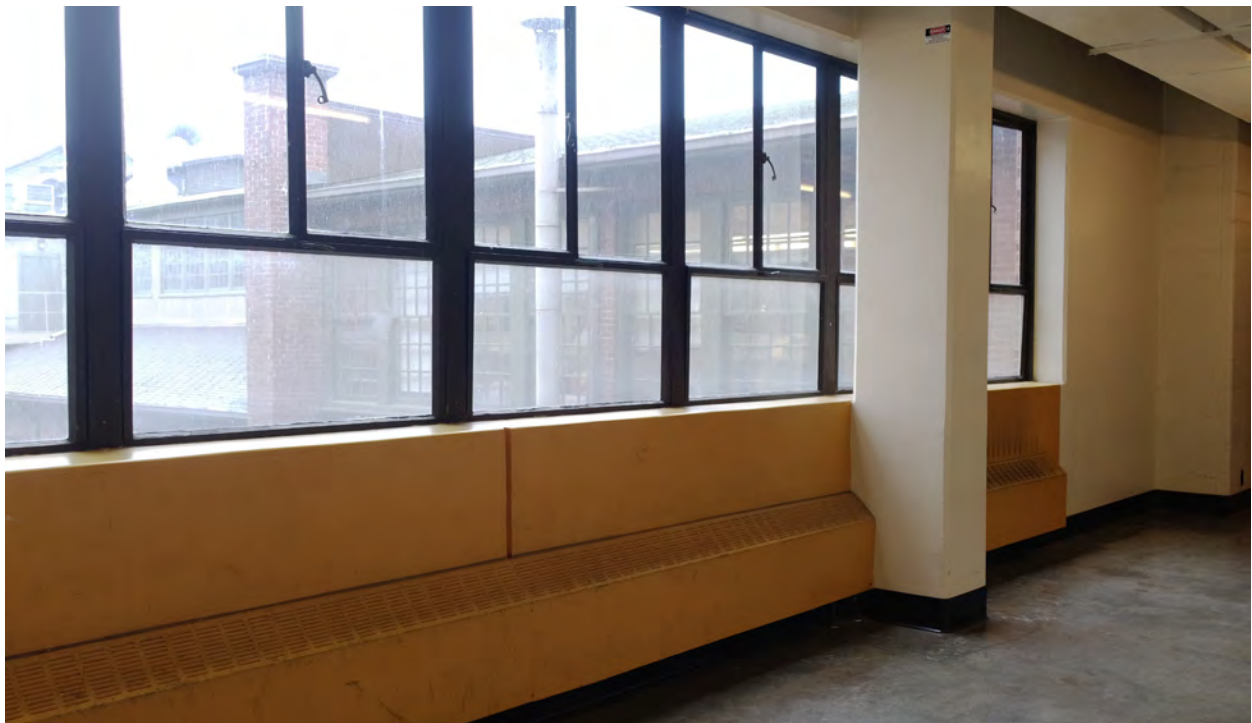
Figure 39. First floor, southeast wing corridor, windows.
