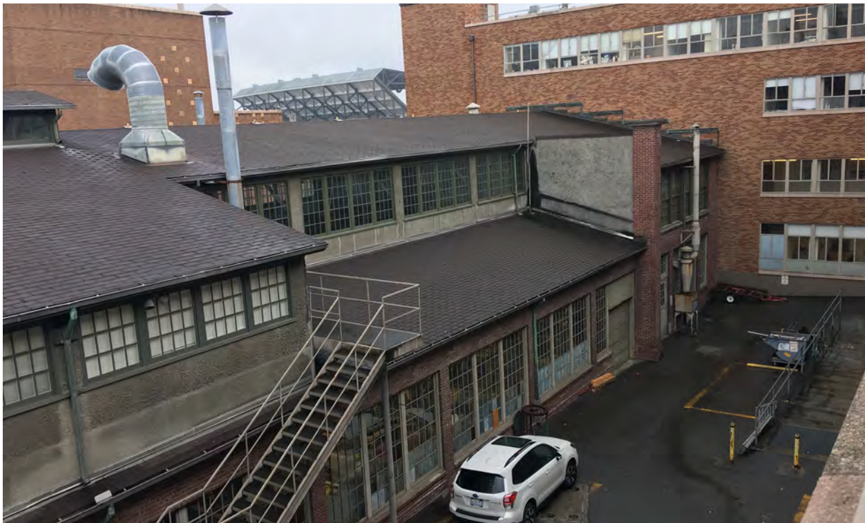
Figure 24. View looking southeast from the Mechanical Engineering building roof of the Engineering Annex connection to the Mechanical Engineering building.
