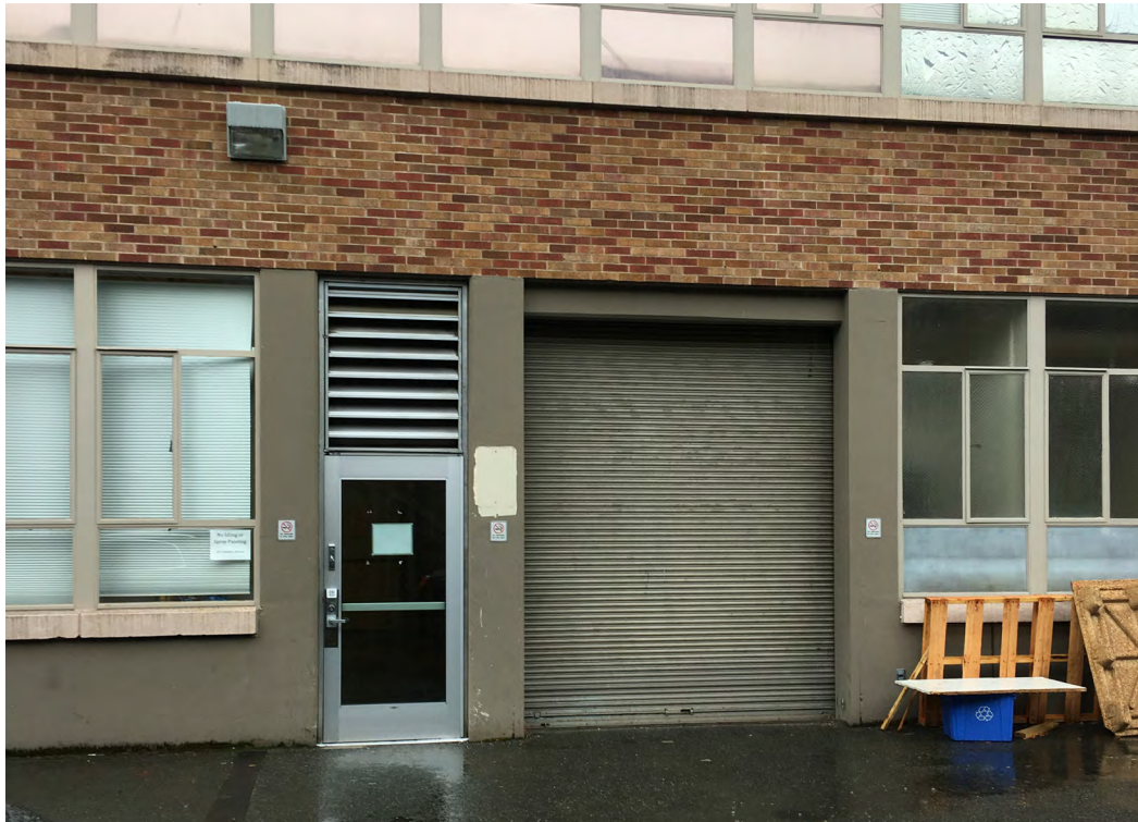
Figure 28. Ground floor entrance off the west side of the service court space.
