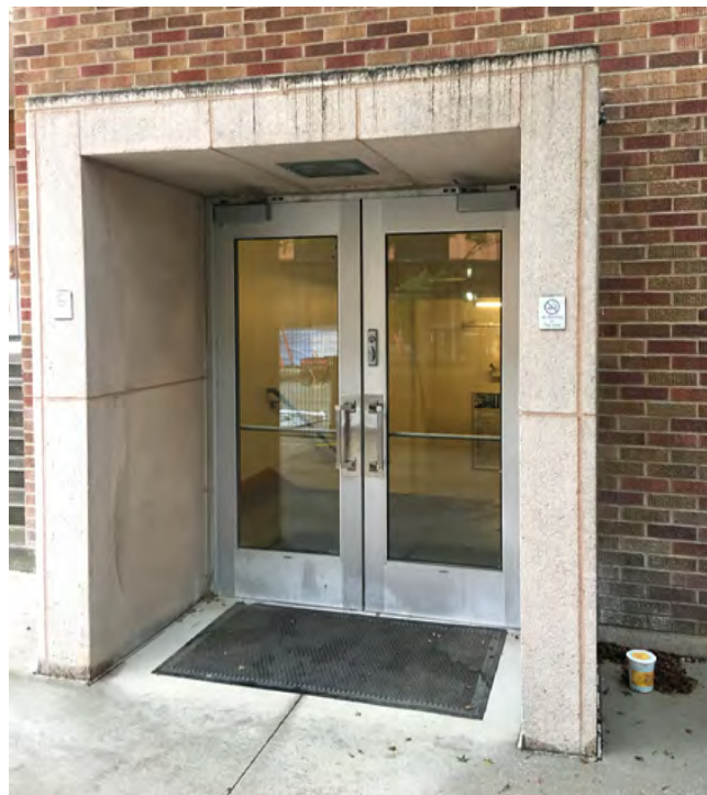
Figure 29. Northwest entrance providing access to the north stairwell.
