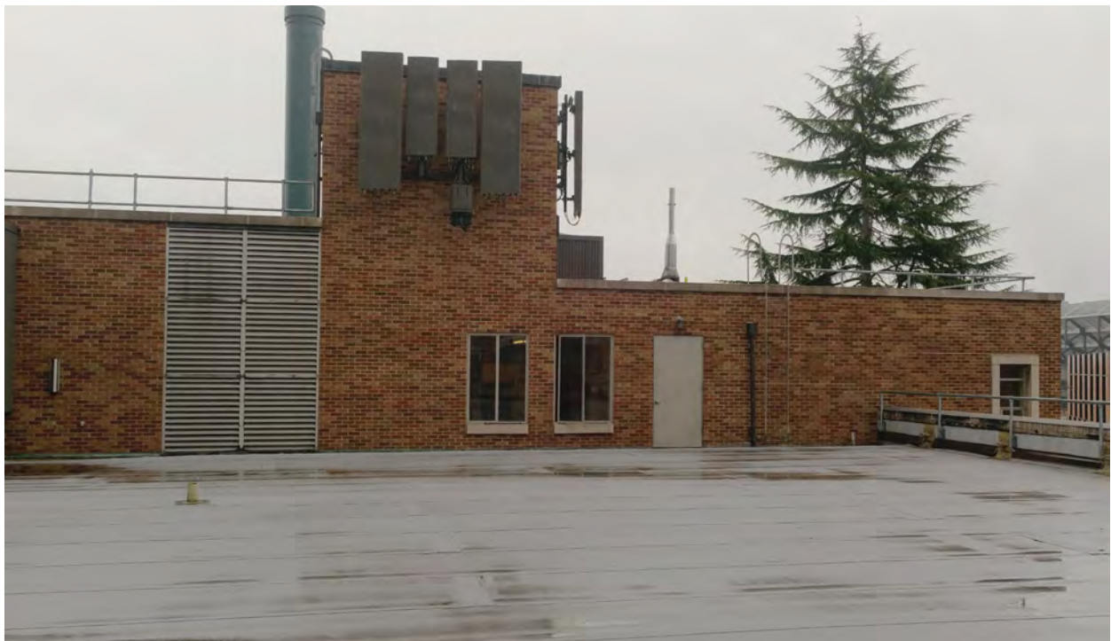
Figure 25. Penthouse and roof, looking east towards the southeast wing.
