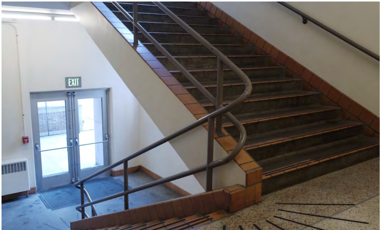
Figure 36. South stairwell looking south from the first floor.
