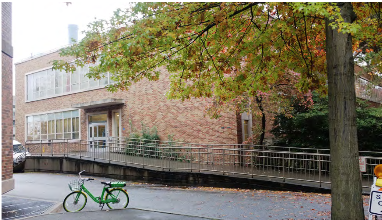
Figure 17. North facade looking southeast with the north entrance in the foreground. This open area and the ramp were reconfigured as part of Loew Hall construction (partly visible at far left in the photograph).
