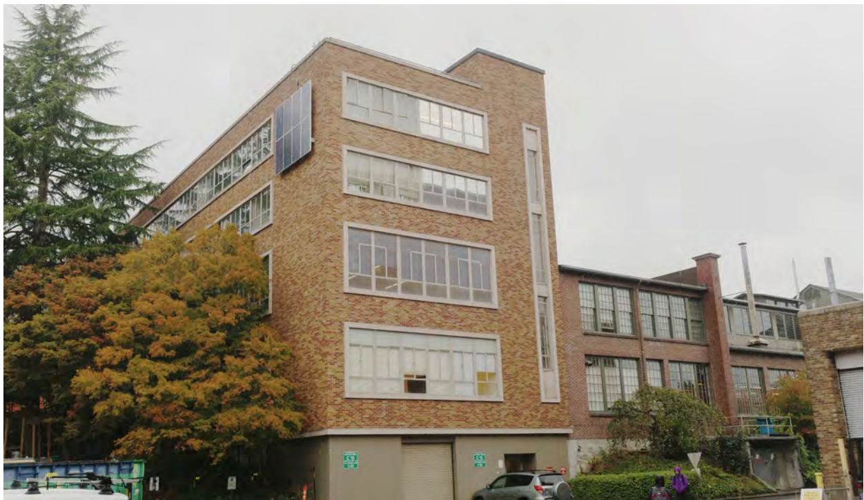
Figure 21. Southeast corner of the building. Note the third story on the southeast wing.
