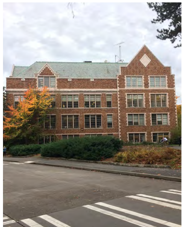
Figure 56. 2016 view of the Communications Building, built 1951. Photograph by Sonja Molchany. Source: WISAARD.
