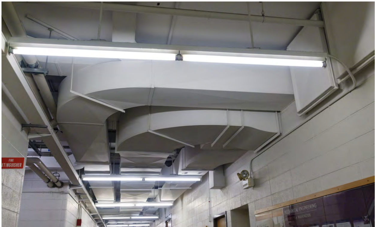
Figure 42. Second floor corridor, typical mechanical equipment.
