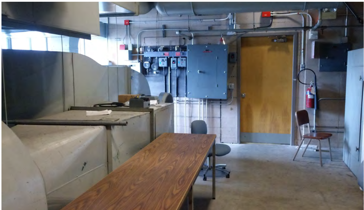
Figure 51. Third floor mechanical room, looking north.
