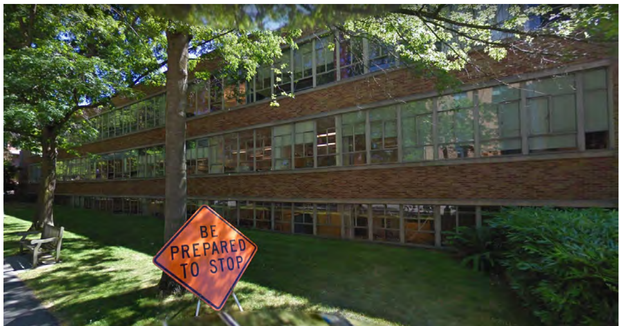
Figure 80. View looking north along the west facade along E Stevens Way NE. Source: Google Street View.
