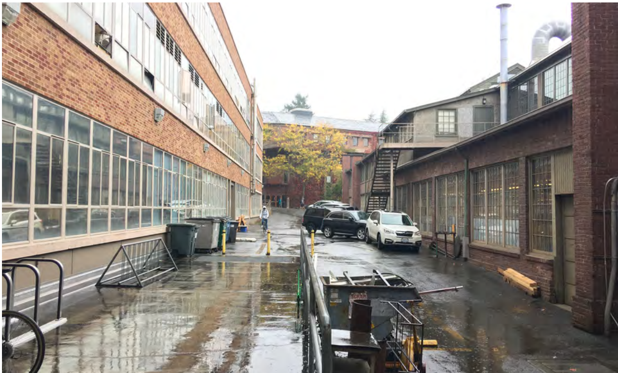
Figure 20. Service court space, looking north. The concrete area in the foreground to the left of the hand railing is the below grade electrical vault.
