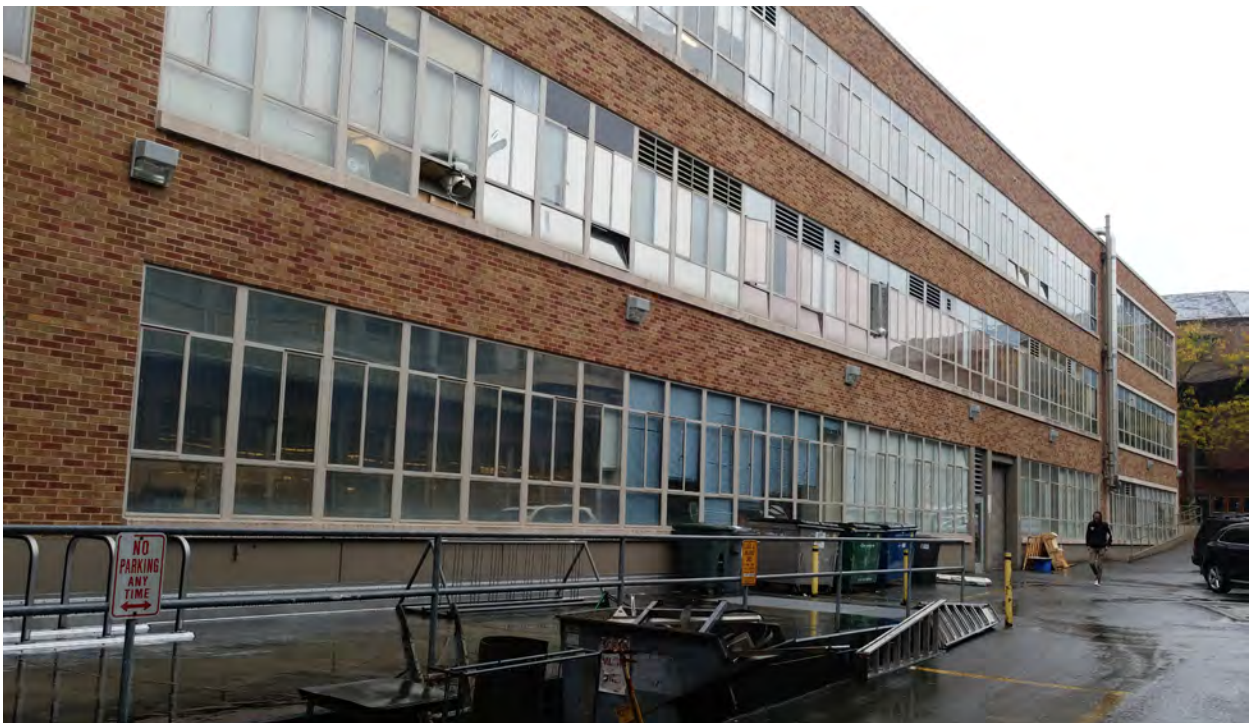
Figure 19. East facade looking northwest along the service court space between MEB and the Engineering Annex.
