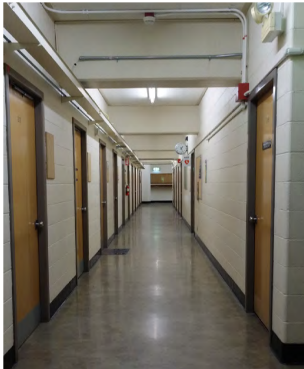
Figure 44. Second floor corridor, southeast wing, looking west.
