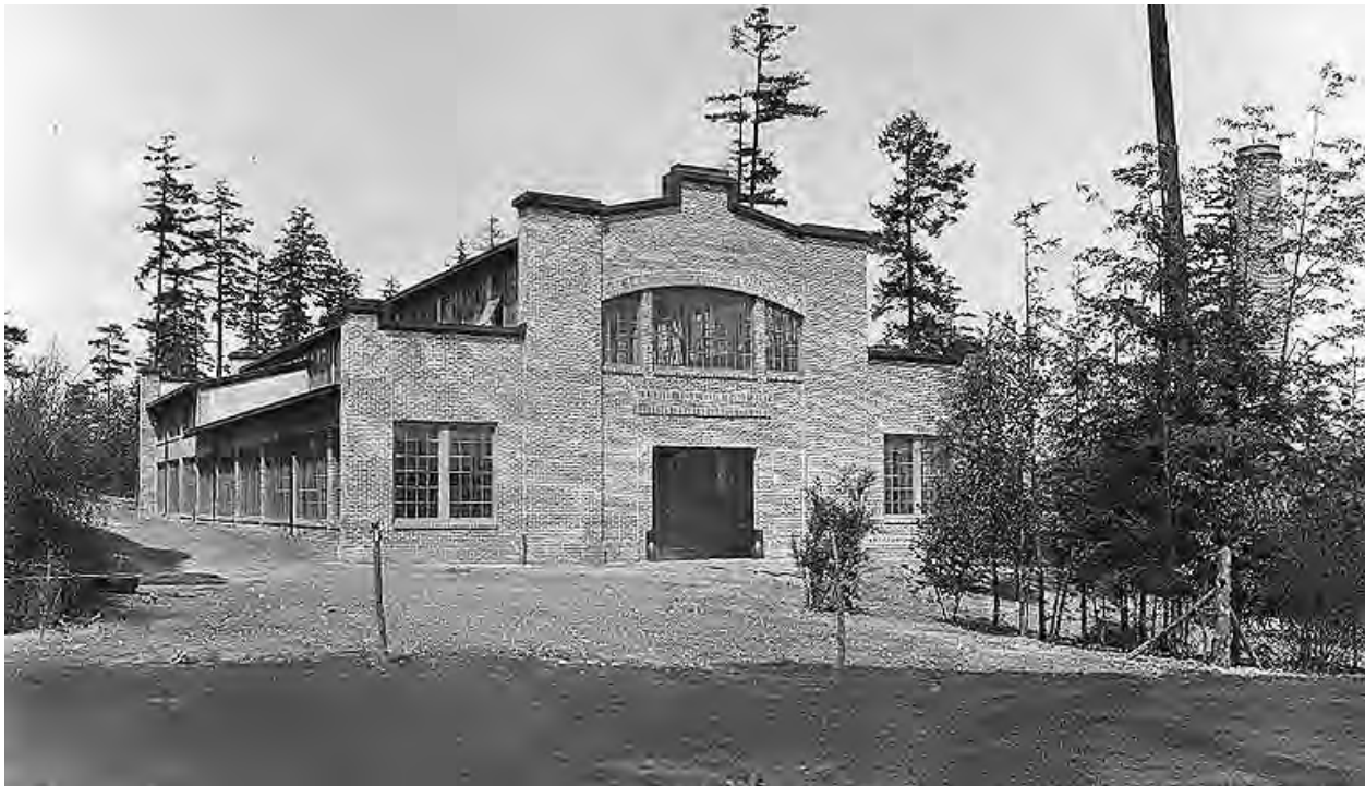
Figure 82. Exterior view and grounds, Foundry Building, 1909. Photographed by Frank H. Nowell. University of Washington Libraries, Special Collections, Negative Number UW17235.
