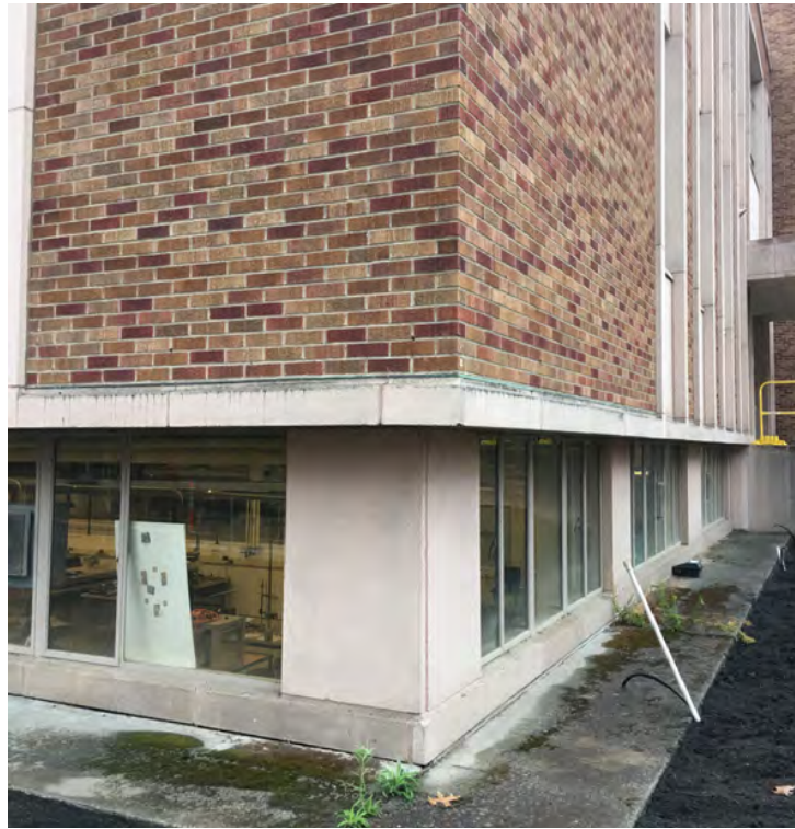
Figure 30. Southwest corner showing the piers at the ground story level with the first story floating above.
