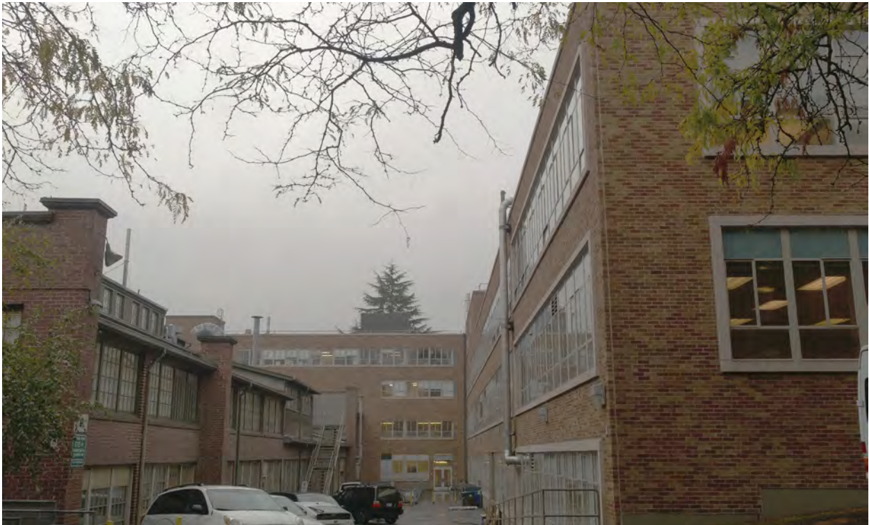
Figure 18. Service court space between the Engineering Annex (left) and MEB (right), looking south.
