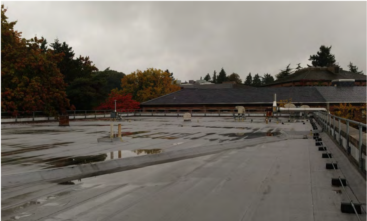
Figure 26. Main roof looking north.
