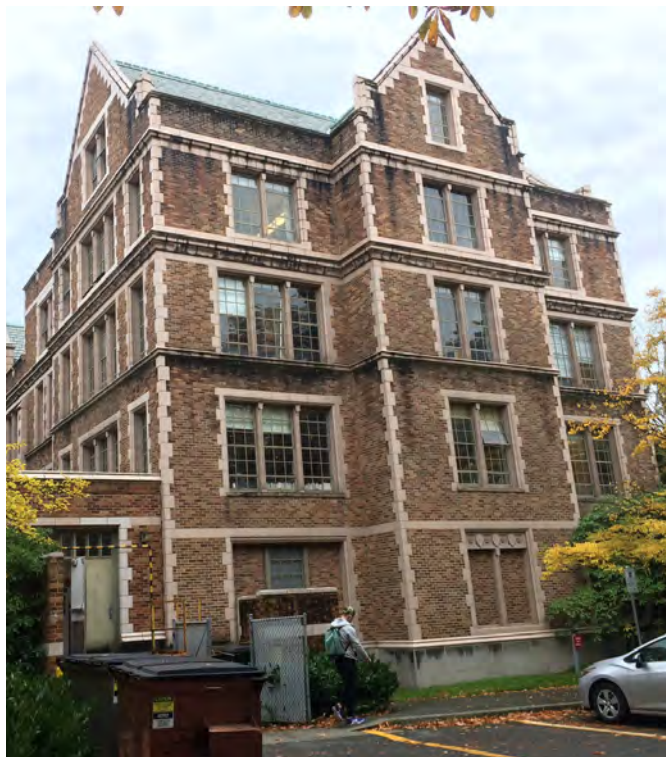
Figure 55. 2016 view of Thomson Hall, built 1948. Photograph by Sonja Molchany. Source: WISAARD.
