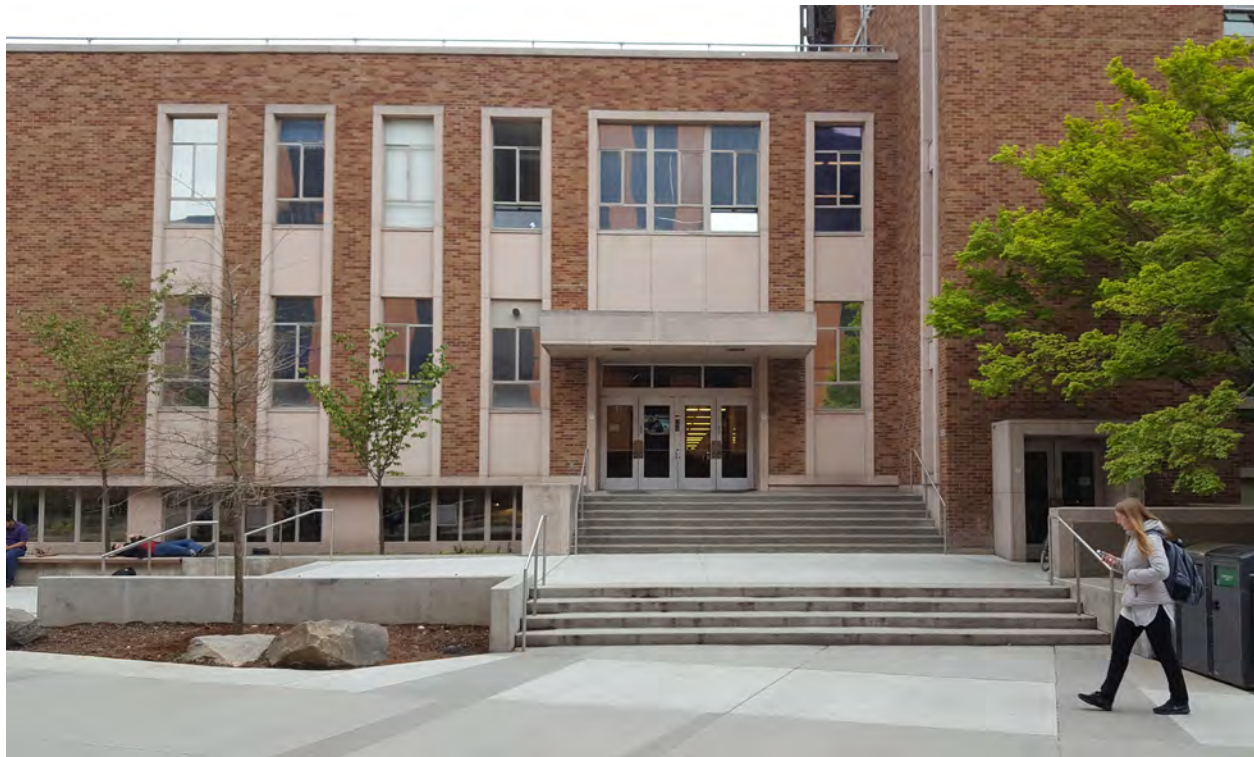
Figure 79. Main entrance on the south facade of the southwest corner block.
